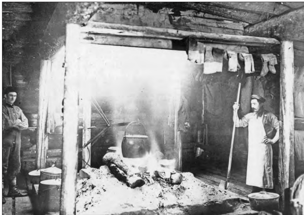
Figure 3. Camboose in a shanty, with rocks and sand surrounded by beams, and showing a bean hole in the foreground. Charles Macnamara collection, Ontario Archives. Used with permission.
